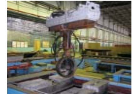
Reserve propulsor system
